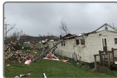
Tornado damage in West Virginia in April. Credit: NWS Charleston, WV
