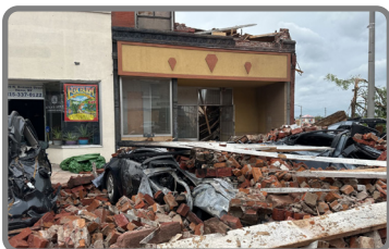
Tornado damage in Rome, NY.
