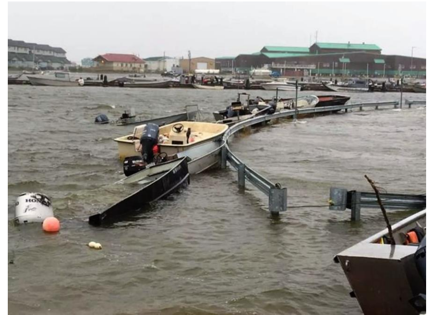
Photo: Kotzebue flooding on October 22, 2024. Credit: Northwest Arctic Borough Emergency Management
